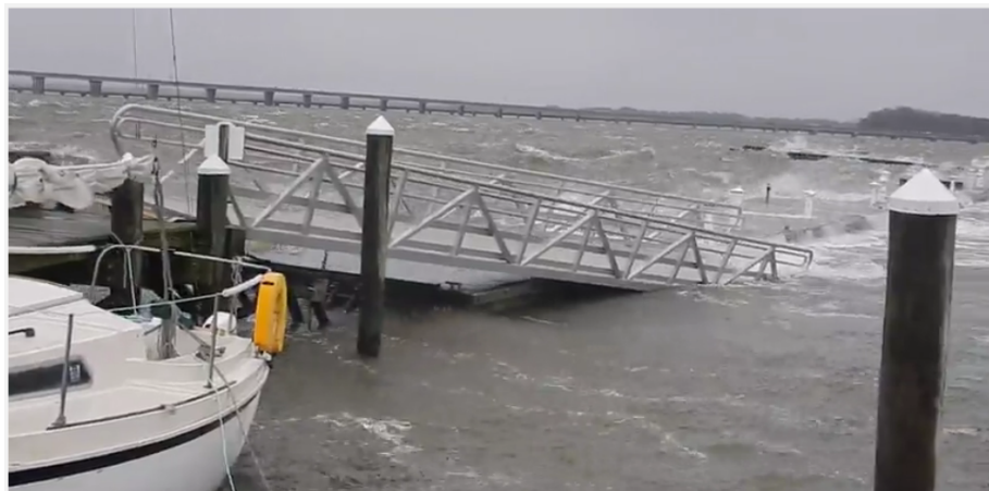
Figure 2. Wave action is strong enough to dislodge the catwalk from the floating pier.
