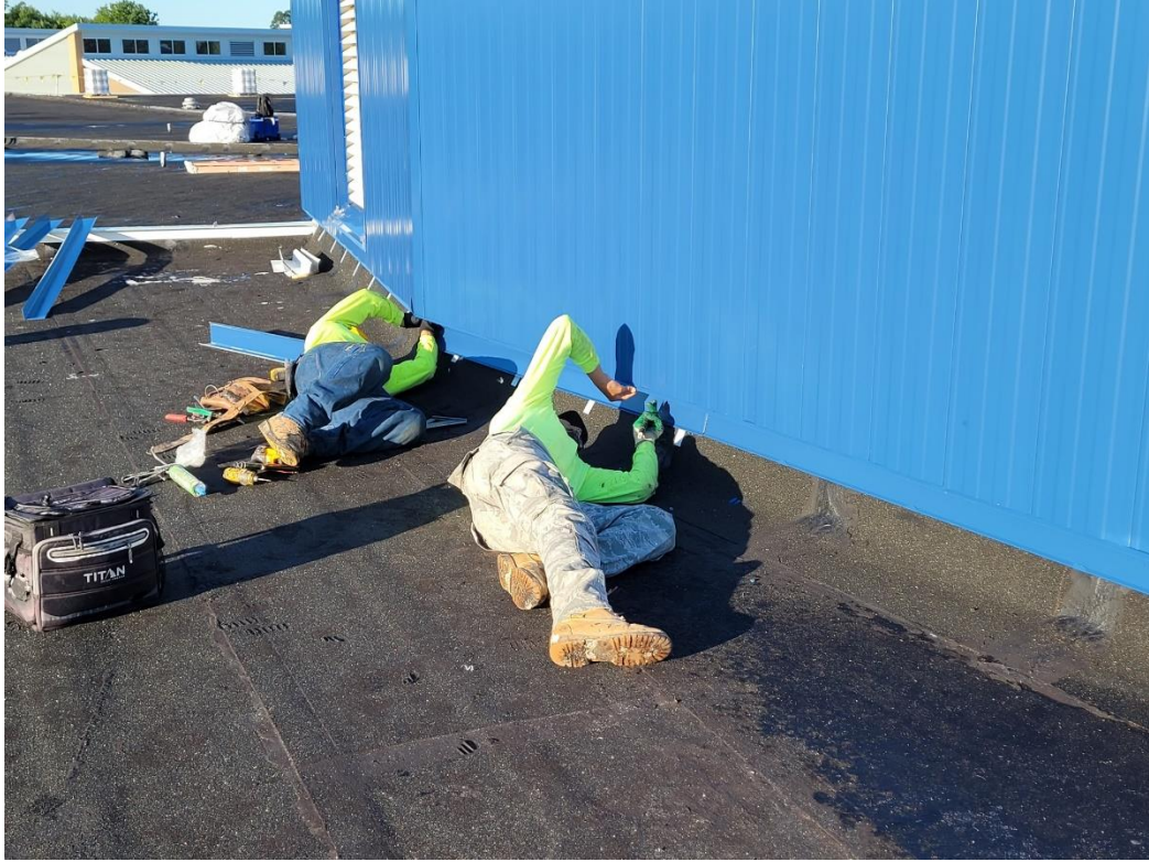
Trimming out Vertical Metal Work.
