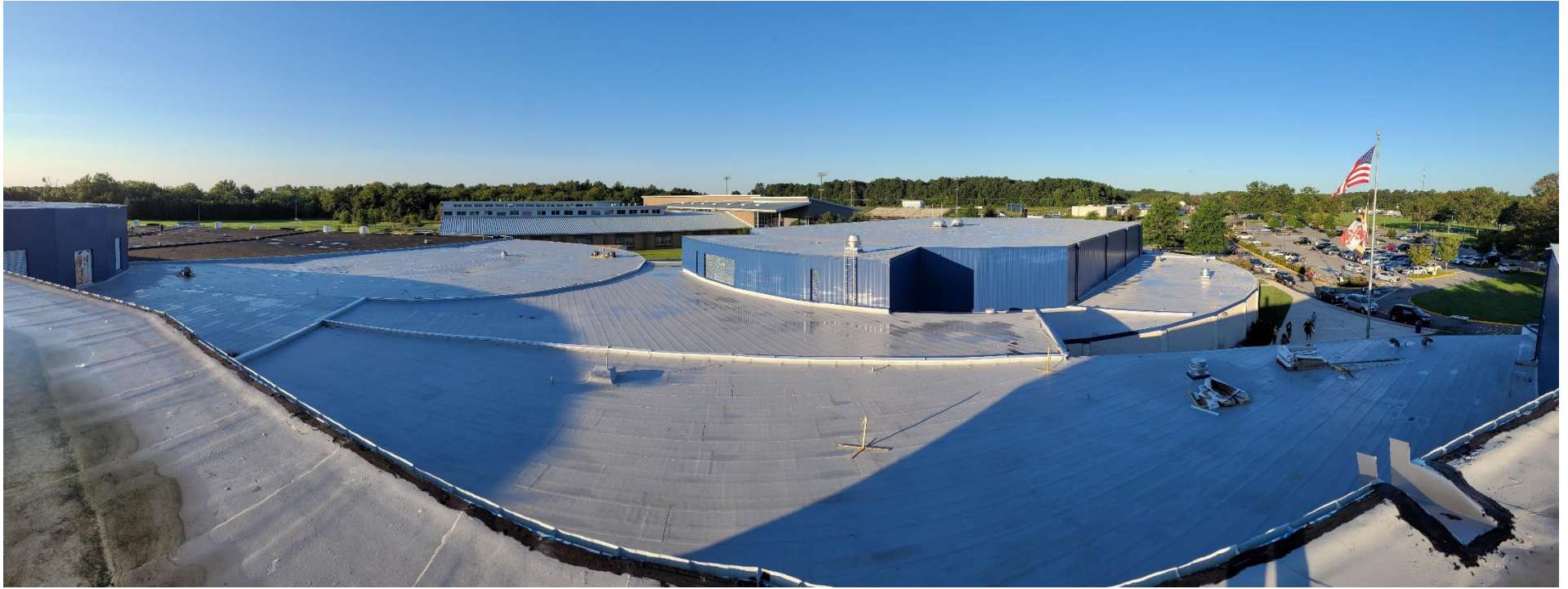
New roof at gymnasium, administration and classroom areas.
