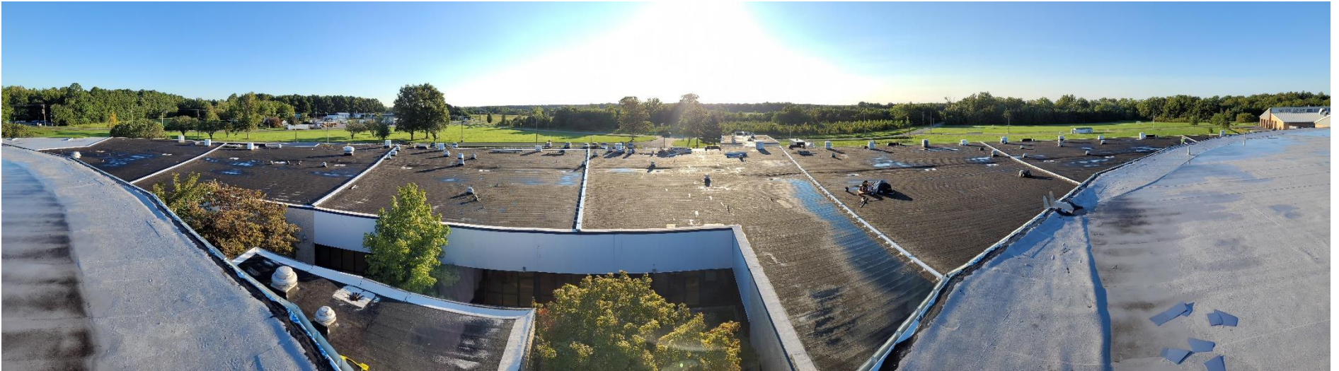
Phase 2 New Roof Southeast Classrooms Complete
