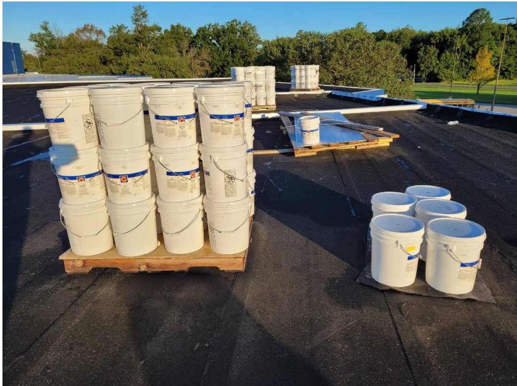
Last Step-Roll on Pyramic Coatic after 60 day cure.
