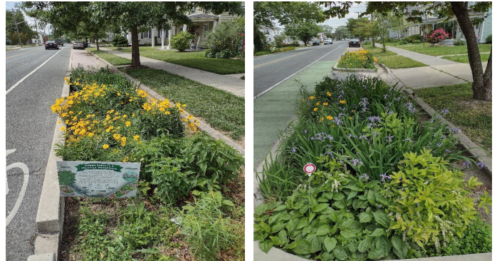
Maryland Ave Curb Bump-outs
