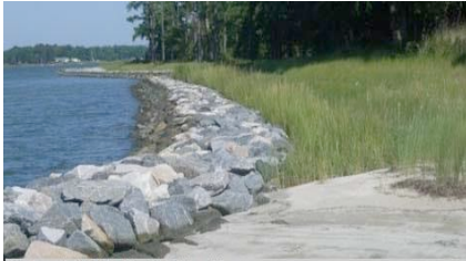
Revetment with Sill & Marsh. Retrieved from https://www.vims.edu/research/departments/physical/programs/ssp/shoreline_management/shoreline_protection/structural_options/index.php . Photo by Shoreline Studies Program
