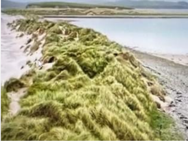
Engineered Dune Rock Core Survives Superstorm Sandy in Bayhead NJ
