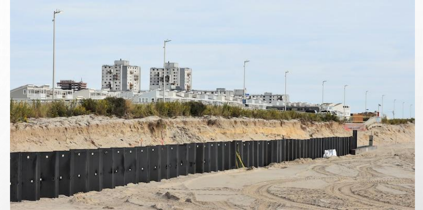
USACE Rockaway Beach NY, Sheet Pile Reinforced Sand Dune Atlantic Ocean Dec 2022
